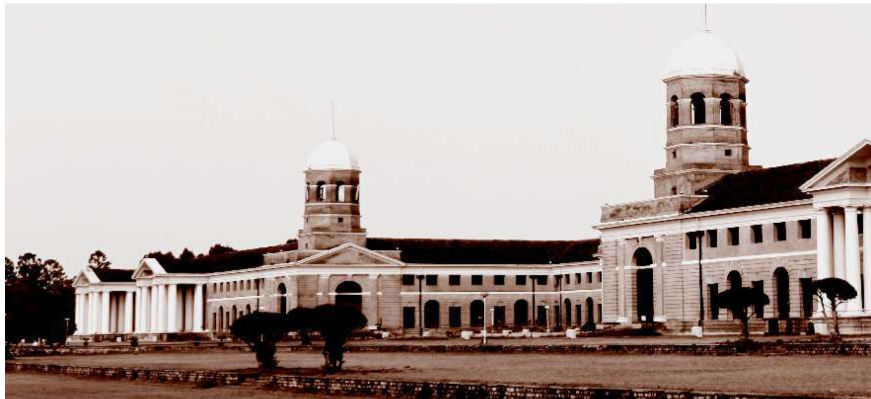
Styled in Greco Roman Architecture by C.G. Bloomfield, the main building was inaugurated in 1929 by then Viceroy Freeman Freeman-Thomas, 1st Marquess of Willingdon. It is now a National Heritage site.
