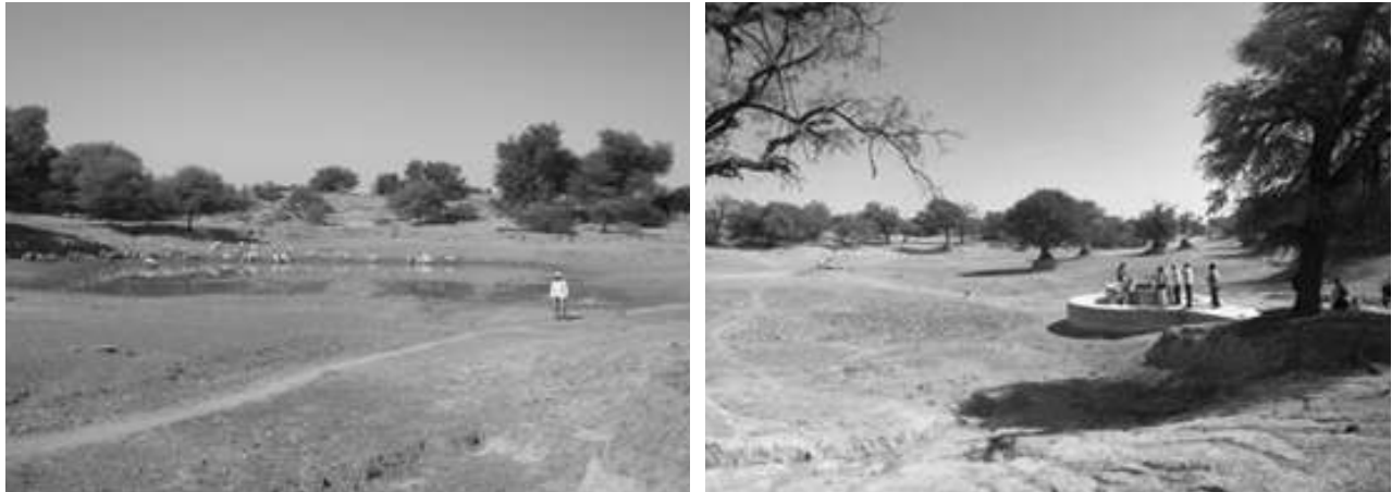
Fig 3.2. Nadi (left) and Kuan in a Talab bed (right) –rainwater harvesting devices in dry areas of western Rajasthan.
